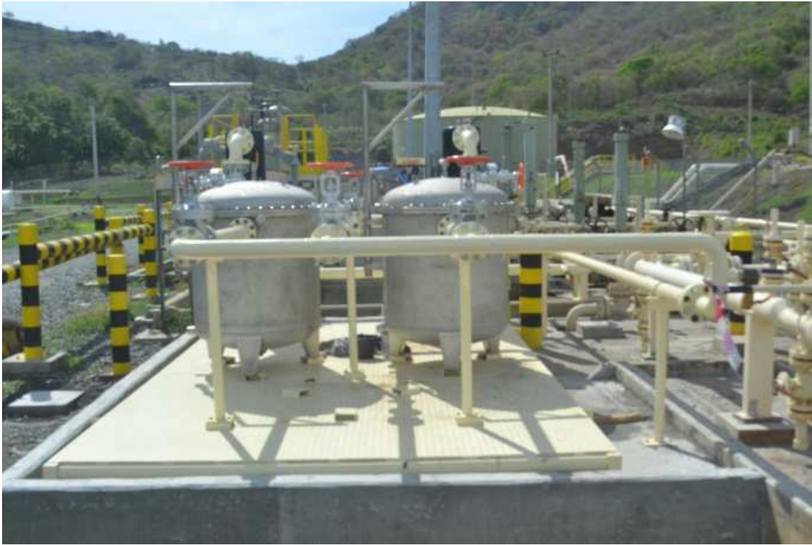
2 x FB 1000/900/32 with a filtering capacity of each 76,000ltr/hr Filter insert change per FB housing after 16 000 000 ltr. ISO 17/11/9
