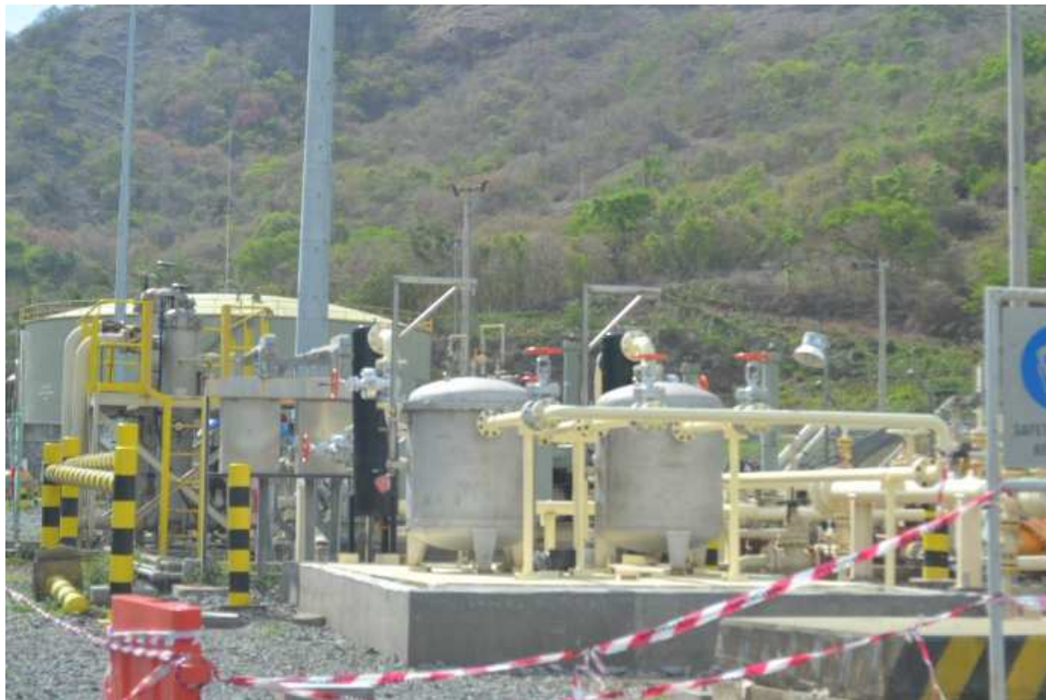
High Flow filter inserts HF 900 changing after 16 000 000 ltr.
