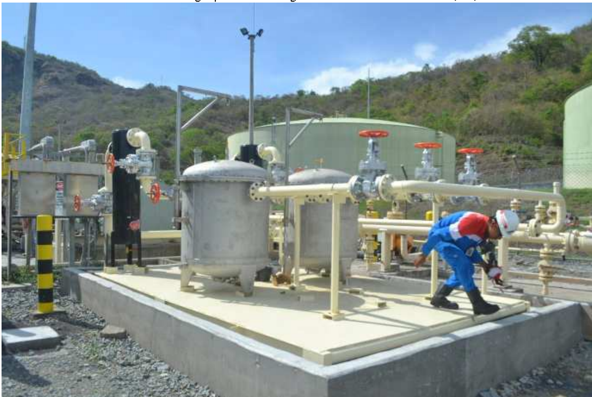
2 x FB 1000/900/32 with a filtering capacity of each 76,000ltr/hr Filter insert change per FB housing after 16 000 000 ltr. ISO 17/11/9
