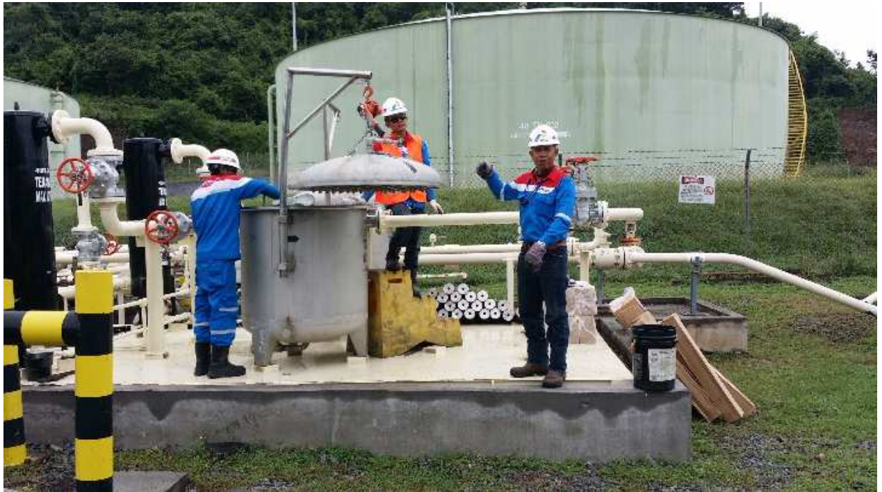
High Flow filter inserts HF 900 changing after 16 000 000 ltr.
