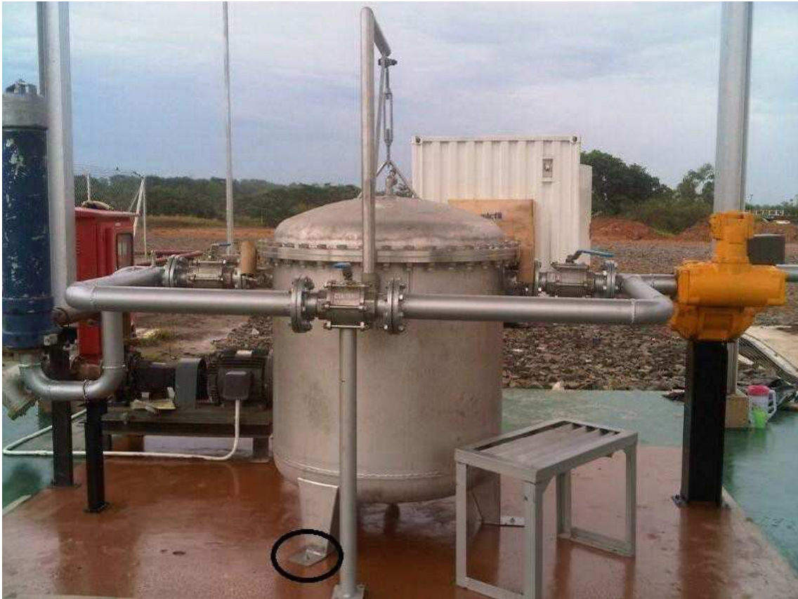
FB 1000/900/32 with FE 900 water block inserts
