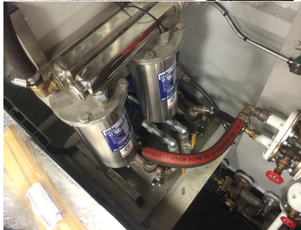
micfil Fuel transfer system with two special pumps and controle box
